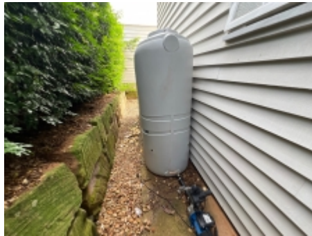
Stored goods should be moved away from the building so as not to hinder visual inspection zone's.
