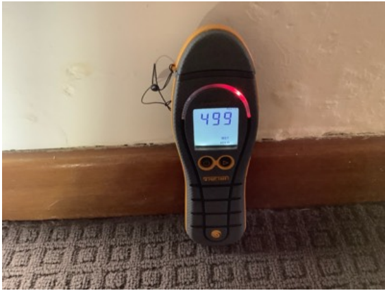
49% moisture detected to the Lounge Room wall.
