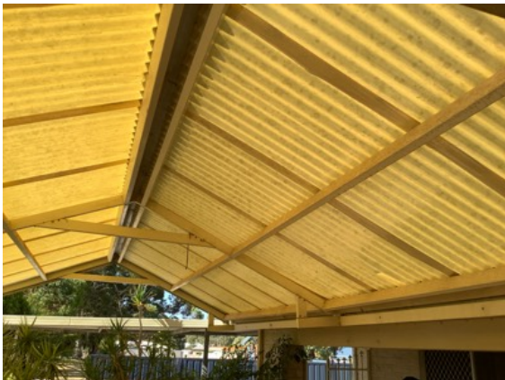
West elevation Patio structure.
