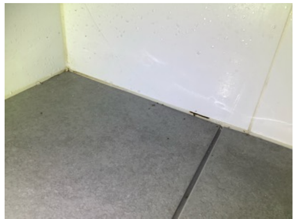
Deterioration/worn grout and sealant joints noted to the Bathroom shower recess floor and wall tiles. Recommend tiler review for repairs and re-seal to waterproof membrane.
