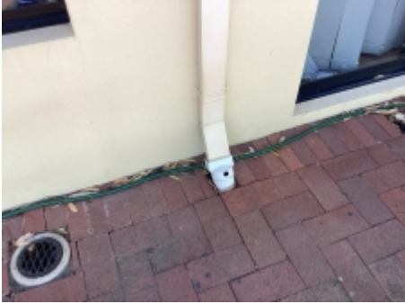
Showing examples of the down pipes
