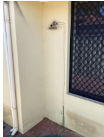
Showing examples of the hot water
