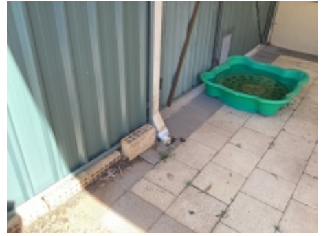
Showing examples of the down pipes
