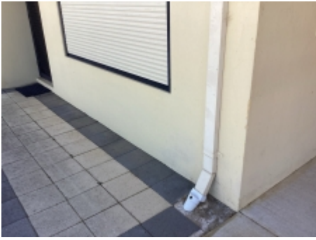
Showing examples of the down pipes
