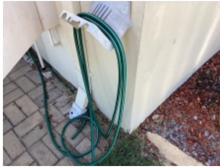
Showing examples of the down pipes
